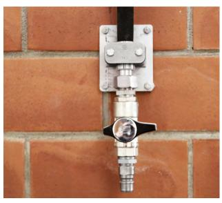
The movable hose is connected to an optimally positioned tap connection. This leads to an effective and cost-saving cleaning because long set-up times are eliminated.
