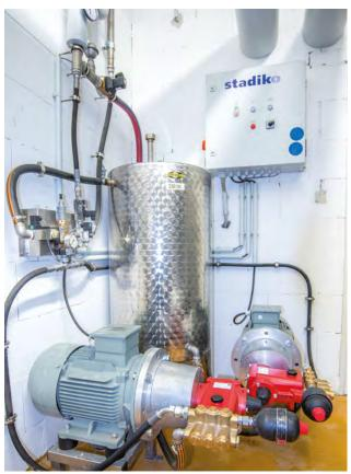
Double-stage system with an external hot water supply
